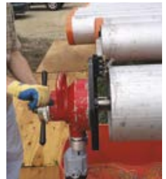
SDB pipe end preparation
